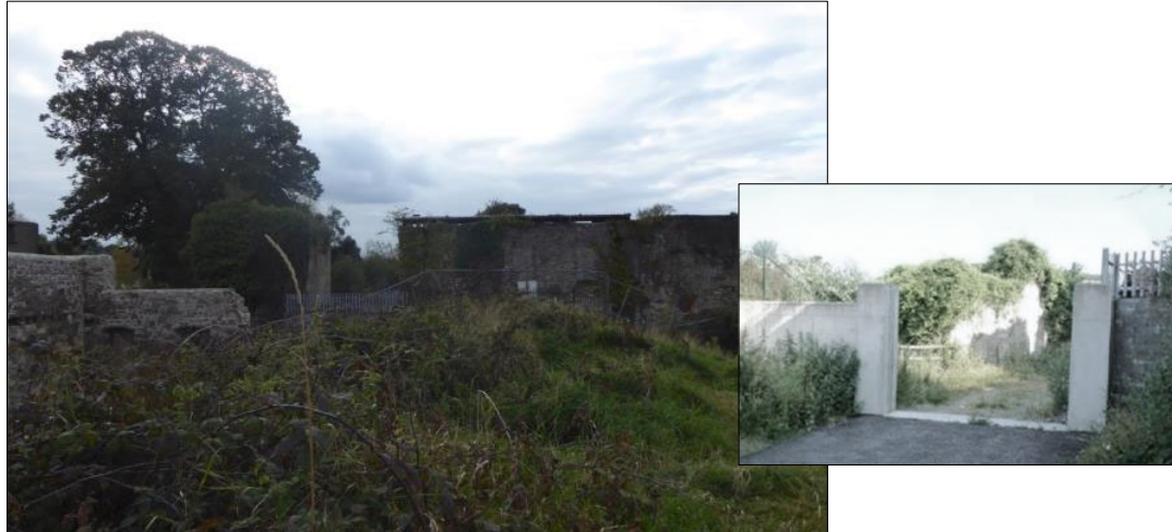
Plate 6 View looking west (from ontop of the berm in the car park) showing the ‘tower’ over grown in ivy and the roofless stores building, (inset: the entrance)
