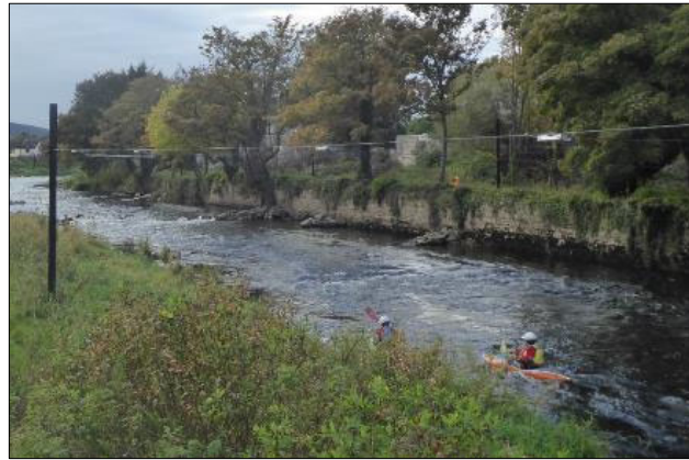
Plate 27 Boundary wall view northwest from the southern banks of the river
