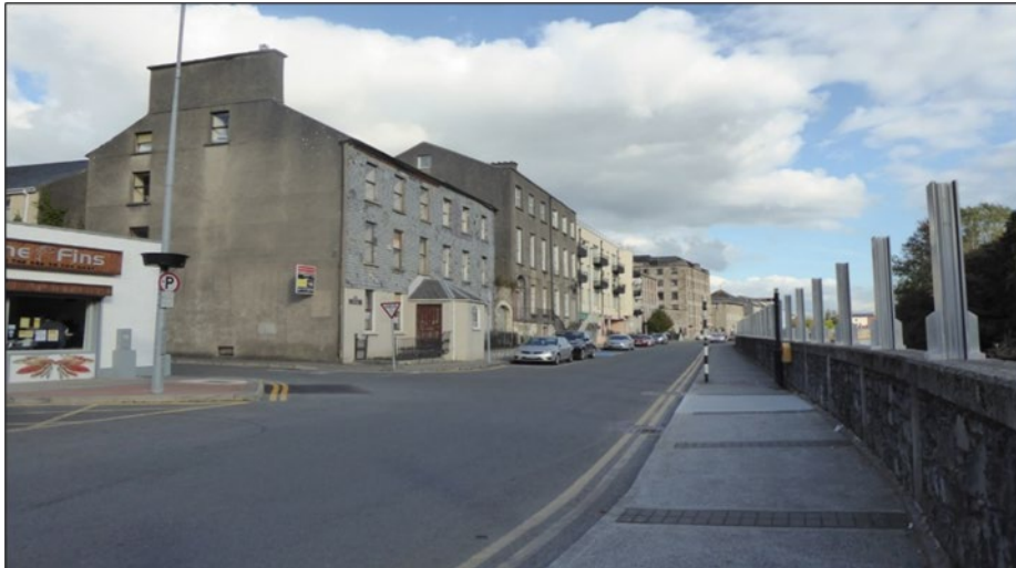
Plate 4 View east along New Quay of RPS 188, 189, 190, flood wall to the right
