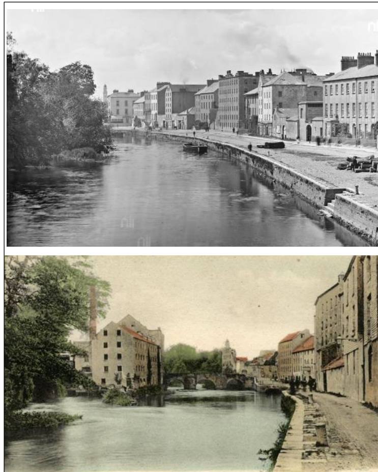
Figure 5 Photographs of Canal Quay Clonmel, view towards Old Bridge (Robert French published between 1880-1900 in the Lawrence Photograph Collection National Library of Ireland) and an early 20 th century colourised photo showing Oldbridge and Hughes Mill – note the narrowness of the Old Quay at this time
