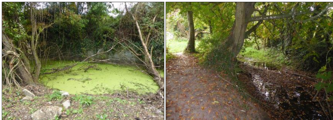
Plate 19 Tail race mid way along its course, it is walled on the northern side
