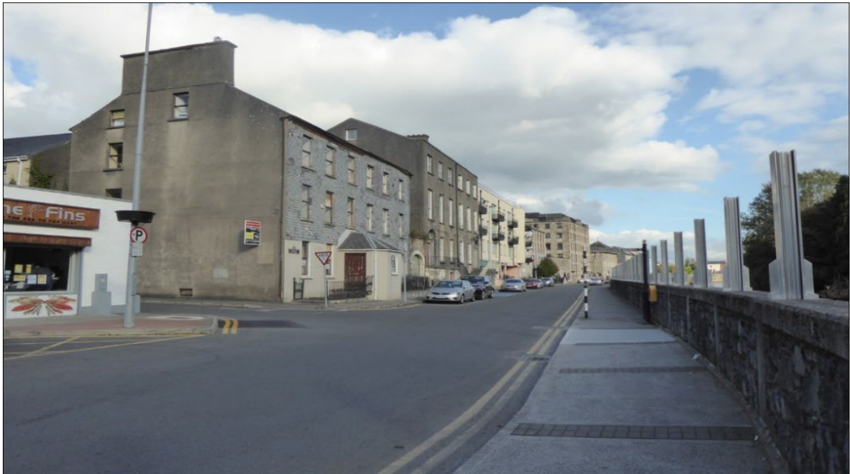
Plate 14-3: View east along New Quay of RPS 188, 189, 190, flood wall to the right
