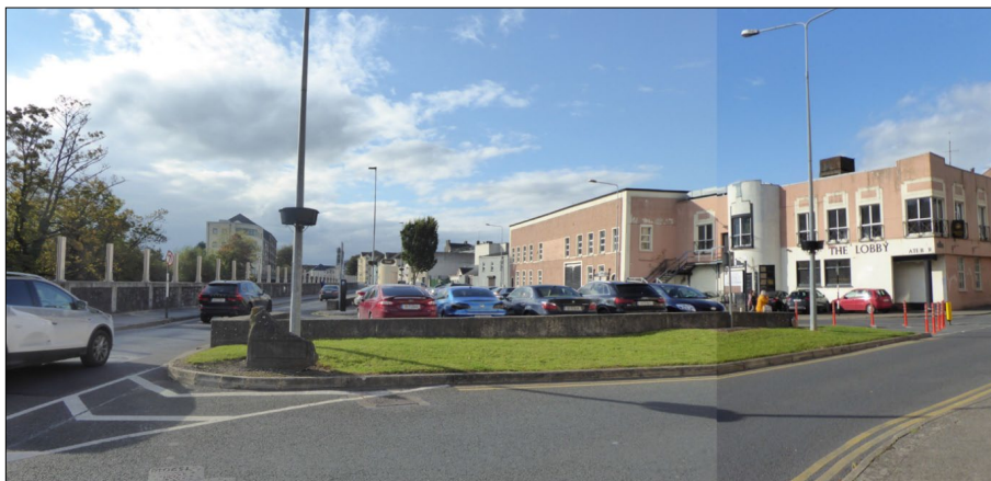
Plate 3 View west of the car park area defined by Quay Street, Old Quay and Sarsfield Street
