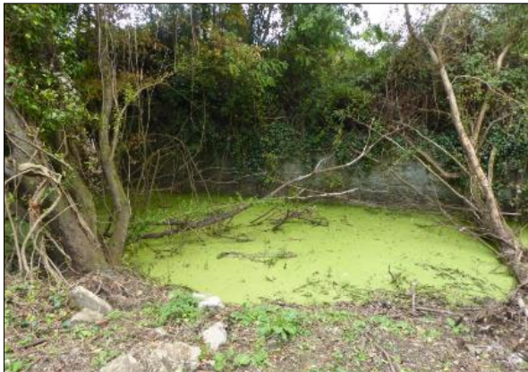
Plate 14-18: Tail race mid-way along its course, it is walled on the northern side (left)
