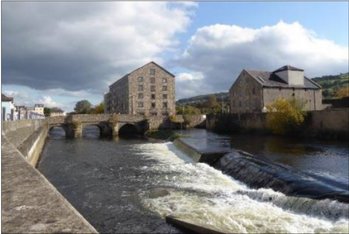
Plate 14-4: Oldbridge (RPS 237, RMP TS083-019002) with new parapets, former Hughes Mill and former Woollen Mill view looking east from the northern banks of the river
