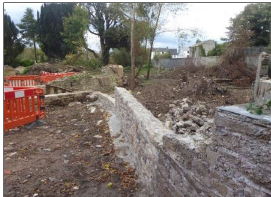
Plate 15 View south of the headrace walls and sluice gate (centre left) to the northwest of Suir Island
