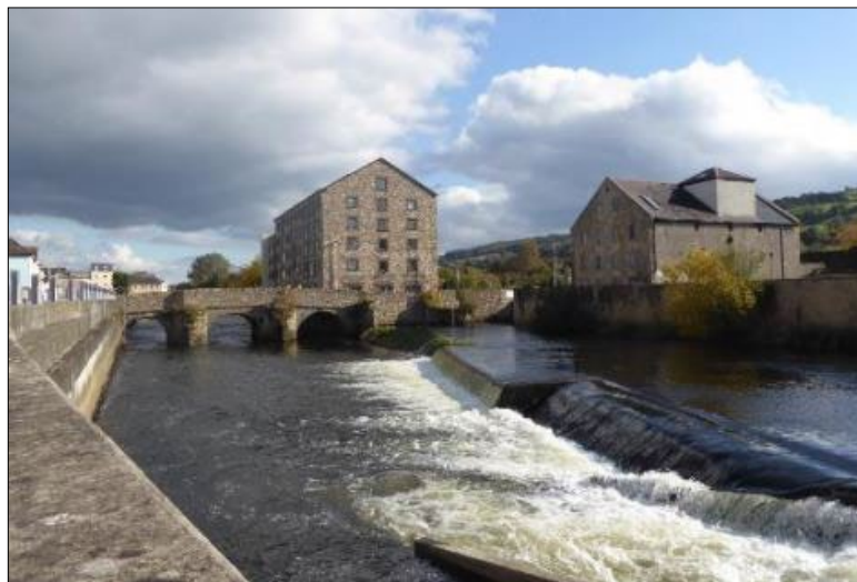
Plate 5 Oldbridge (RPS 237, RMP TS083-019002) with new parapets, former Hughes Mill and former Woollen Mill view looking east from the northern banks of the river
