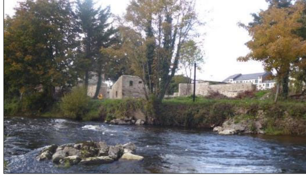
Plate 26 Boundary wall view northwest from the southern banks of the river
