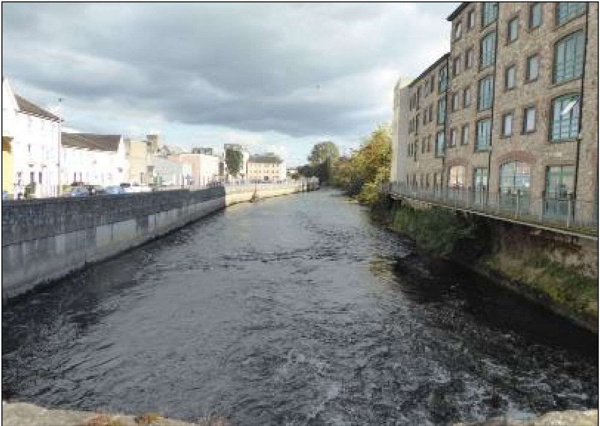
Plate 14-1: View east along the Quays from Old Bridge, restored Hughes mill on Suir Island to the right
