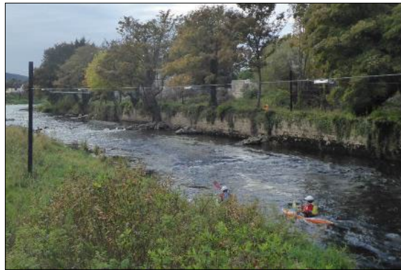
Plate 23 Boundary wall view northwest from the southern banks of the river
