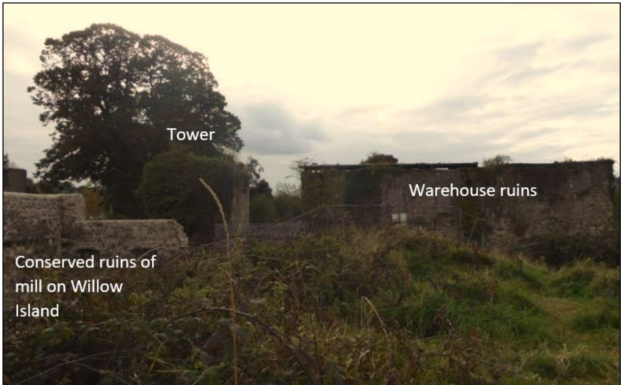
Plate 14-8: View looking west (from on top of the berm in the car park) showing the 'tower' over grown in ivy and the roofless stores building,
